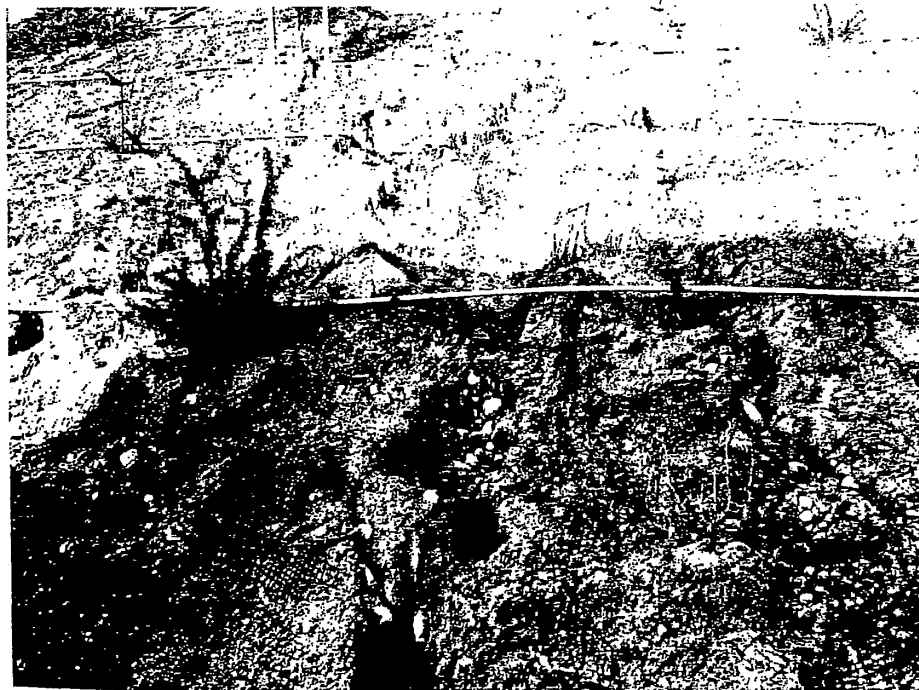
Address: Deputy Jake Drive, Lots 50 & 51 Exterior, overview, ascending 2:1 slope (note surface erosion at several locations; limited to a foot in depth, total slope height is about 50 feet).
