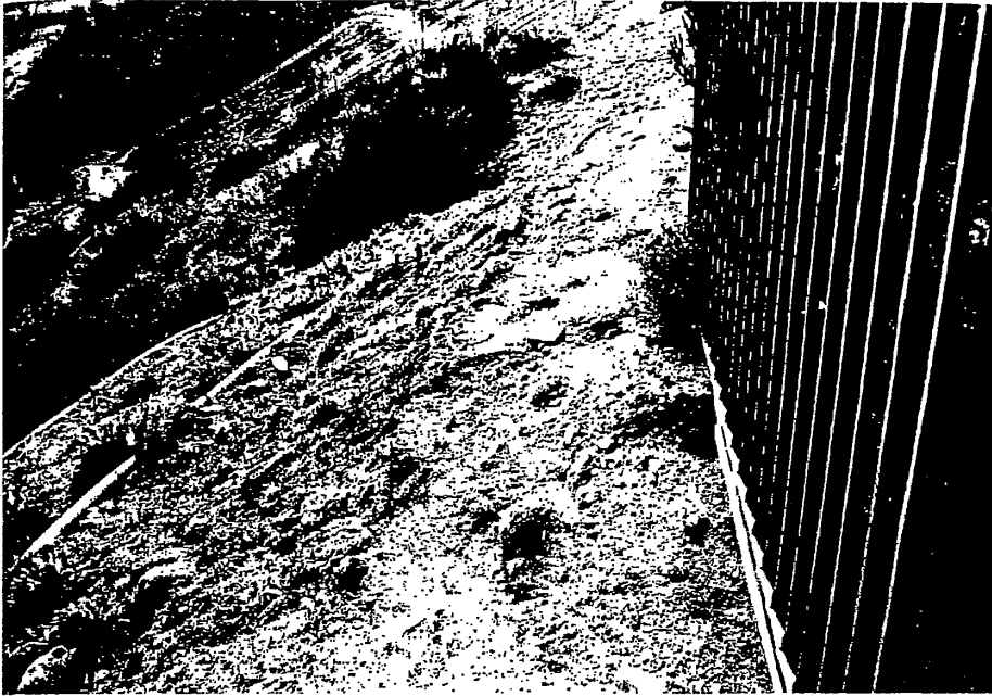
Address: Kirsch Court, Lot 39 Exterior, overview (near top-of-slope; note sloughing and minor ground cracks; also note wet soil conditions and apparent water seepage from the side yard of the home).
