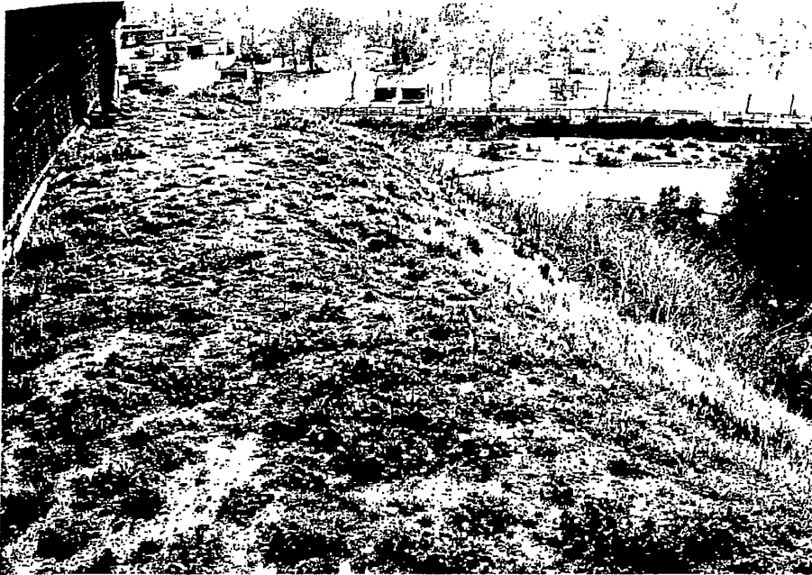
Address: Mathew Place Behind Lots 7-15 Exterior, generally behind Lot#7 (note the soil at the top of the slope is dipping by a few inches, appears to have been affected by localized settlement or slope creep).
