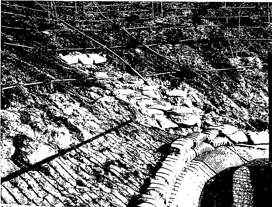
Address: Deputy Jake Drive, Lots 50 & 51 Exterior, overview, ascending 2:1 slope (note surface erosion at several locations; limited to a foot in depth, total slope height is about 50 feet).
