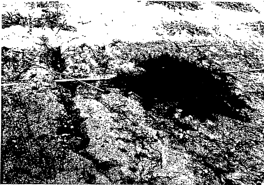
Address: Deputy Jake Drive, Lots 50 & 51 Exterior, overview, ascending 2:1 slope (note surface erosion at several locations; limited to a foot in depth, total slope height is about 50 feet).
