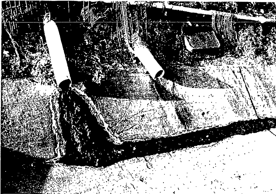
Address: Kirsch Court, Lot 40 Exterior, overview (consistent seepage from the subdrain pipe into V-ditch, east side of Lot #40).
