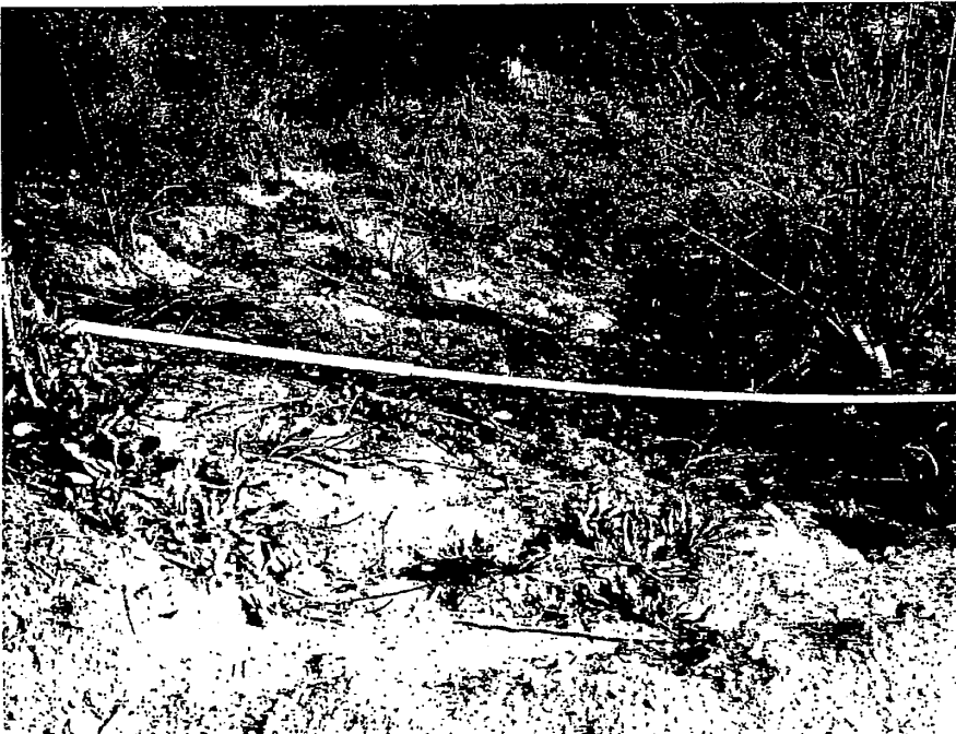
Address: Mathew Place, Lot 16 Exterior, overview, two separate surficial failures on the southerly descending slope behind Lot 16 (the depth of the failure is about 2 to 3 feet located within the upper 15 to 20 feet of the slope).
